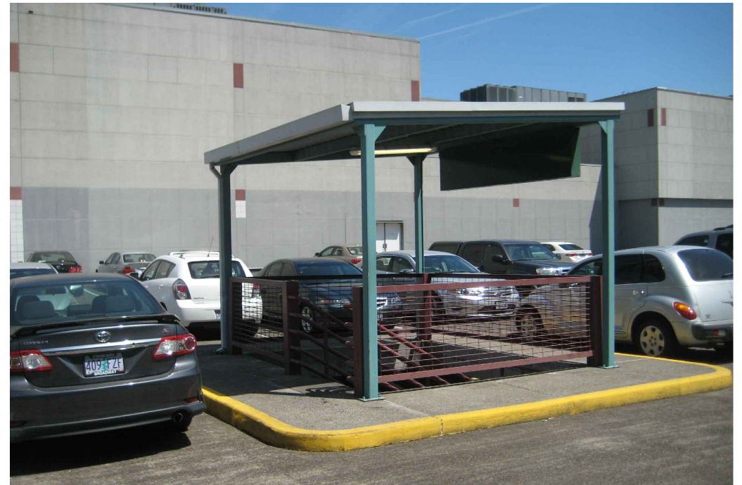
roof structure at existing parking garage stair
