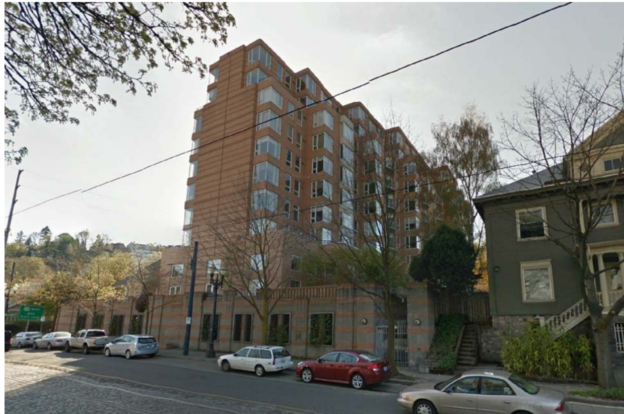
View looking west along SW 18th Avenue towards existing apartment building
