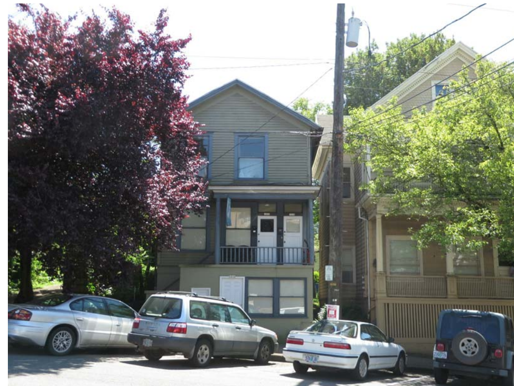
View looking south at adjacent buildings on west property line
