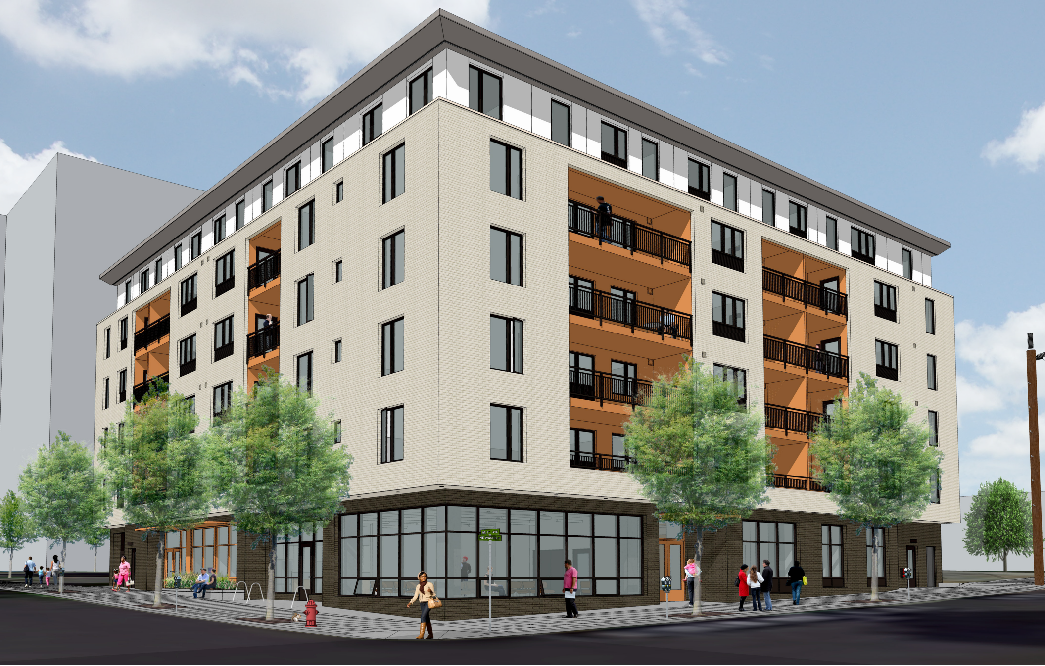
VIEW FROM SOUTHWEST - CURRENT
