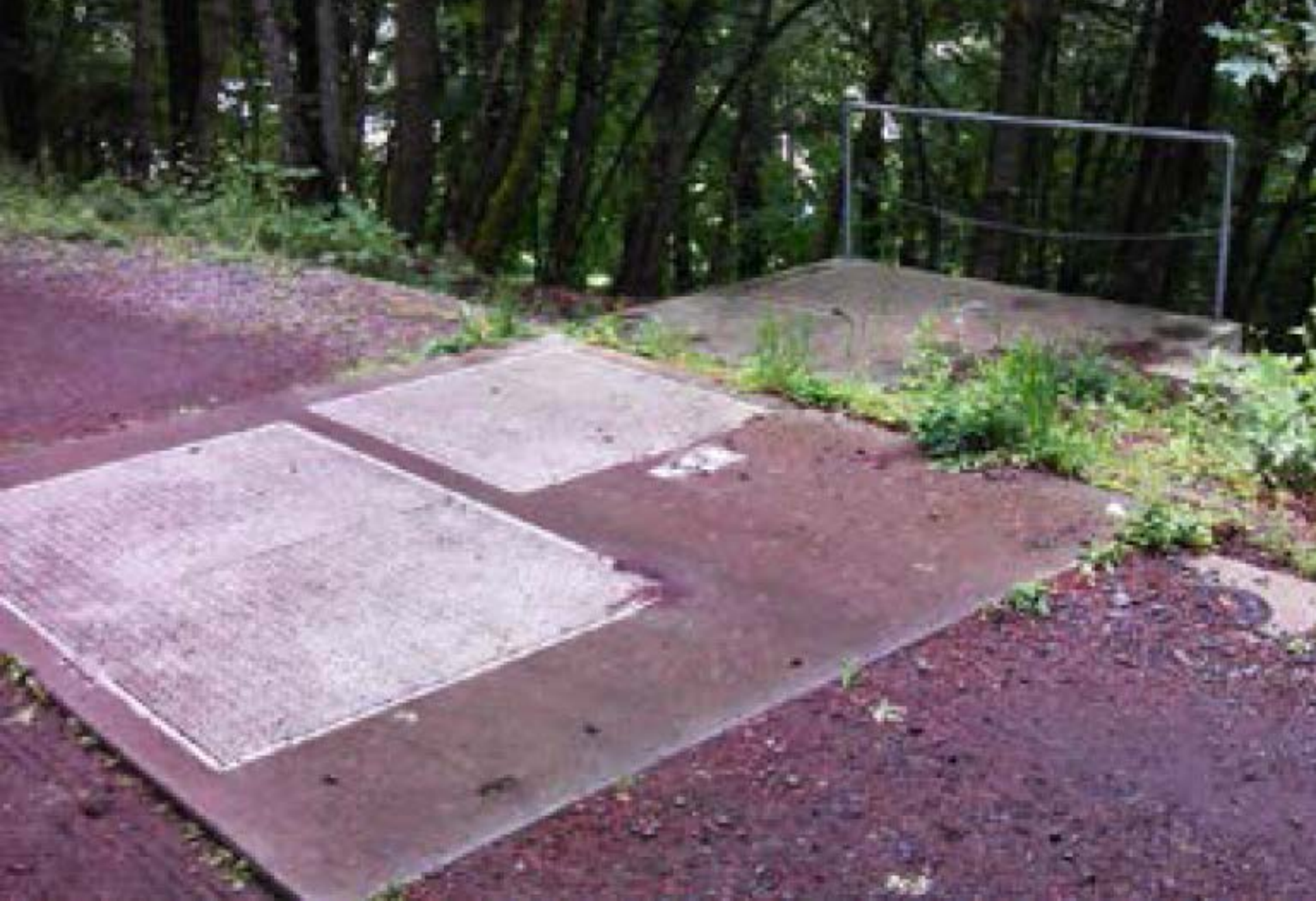
Work Area 6: Existing vault west side SE Reservoir Loop Drive.
