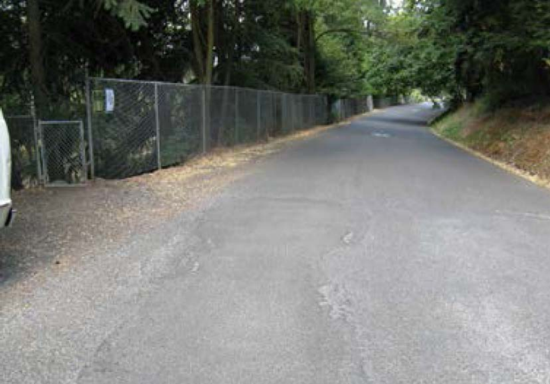
Work Area 3: SE Lincoln Drive through c-zone.
