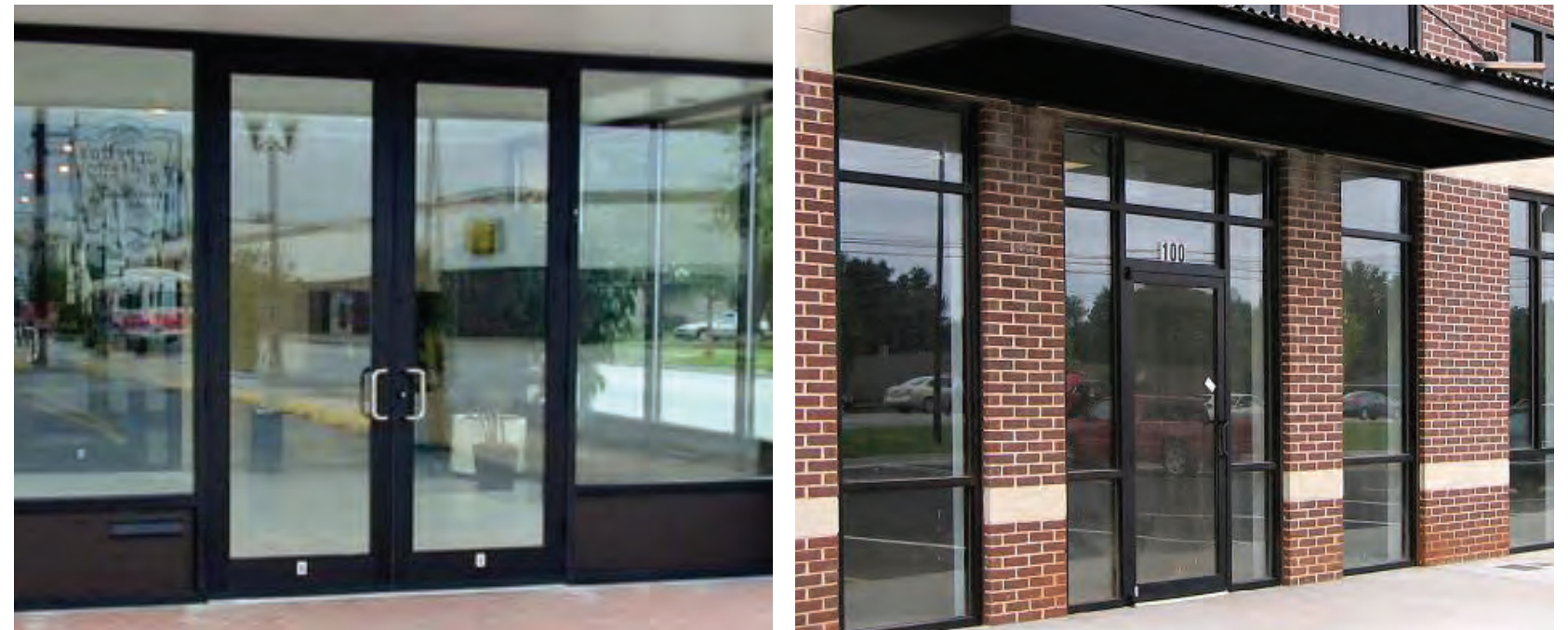
REPRESENTATIVE EXTERIOR IMAGES OF ALUMINUM STOREFRONT
