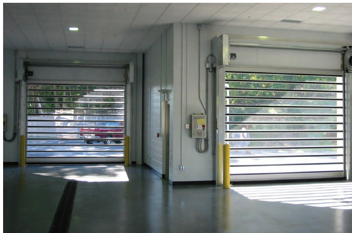
VEHICULAR ENTRY DOOR FROM INTERIOR
