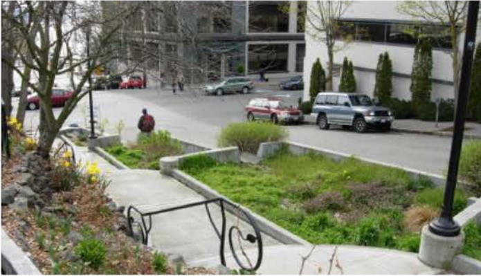
TERRACED CONCRETE STORMWATER PLANTER
