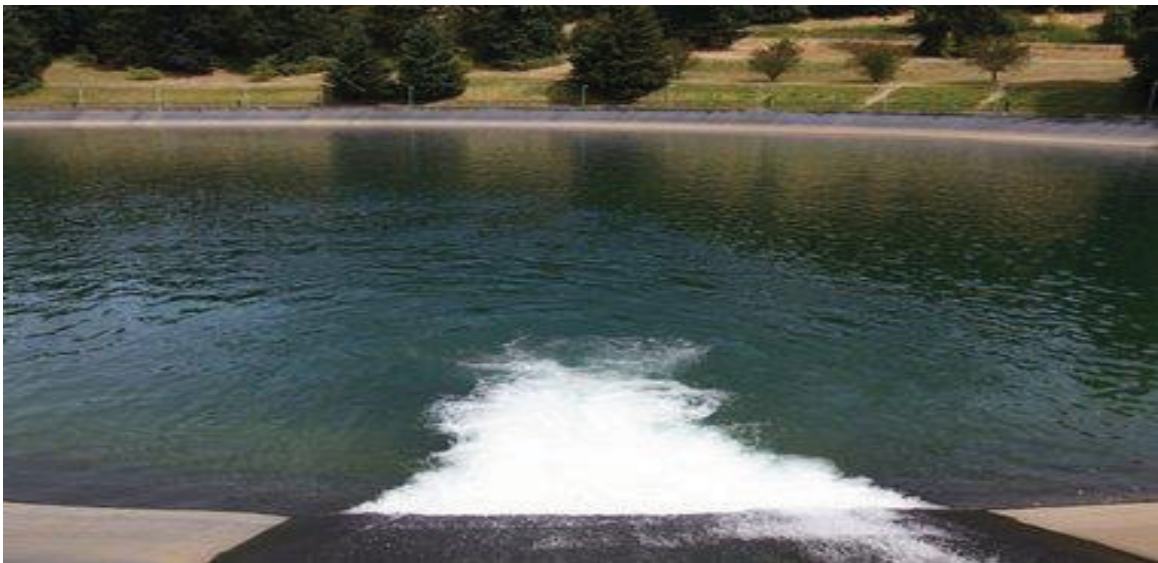
Mt. Tabor Reservoir 5. Open reservoir drinking water inlet: waterfall agitating action aerates water providing oxygen, promotes water movement, while removing unwanted gases. Open reservoir sunlight also provides a public health barrier, using a natural, sustainable, gravity fed carbon-free process delivering safe and healthy water.
