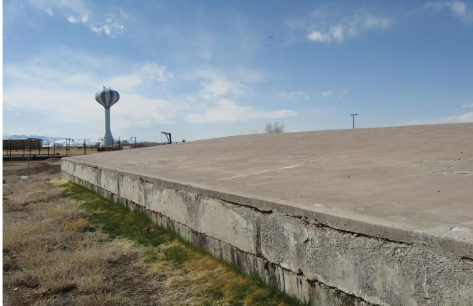
Covered Alamosa, Colorado reservoir where Salmonella bacteria from prolonged bird roosting exposures were not visible or detected, causing illness and death
