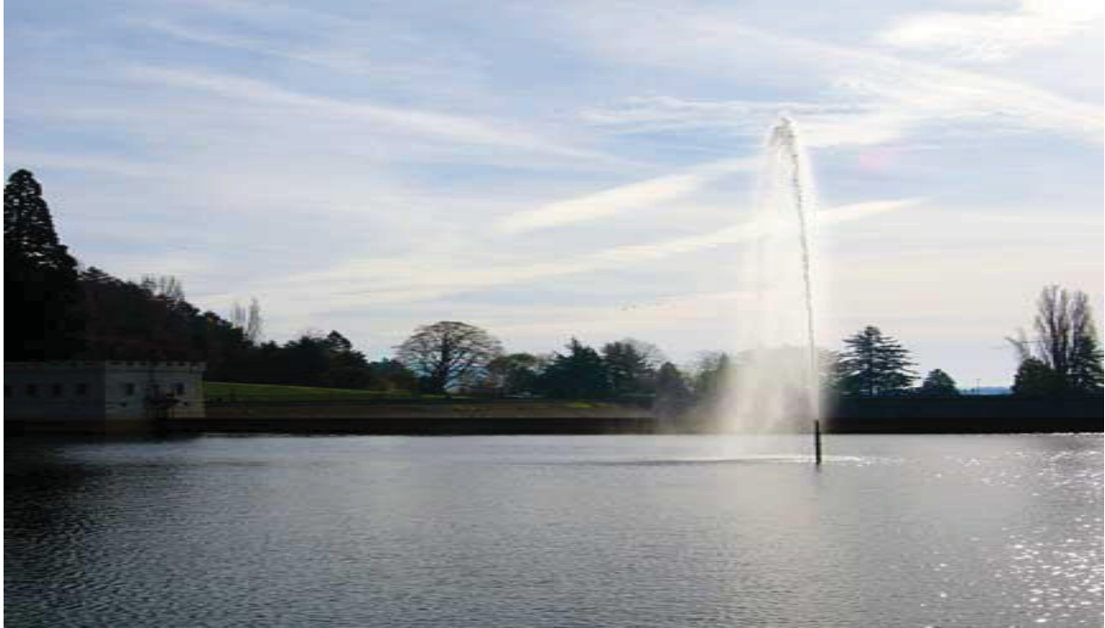
Mt. Tabor Reservoir 6. Open reservoir water oxygenation from fountain and waterfall aeration also removes toxic and carcinogenic gases such as radon and chloroform. Gases escape efficiently through diffusion – the movement of particles from high concentration to lower concentration. Diffusion is enhanced by wind and natural convection in water wave action.
