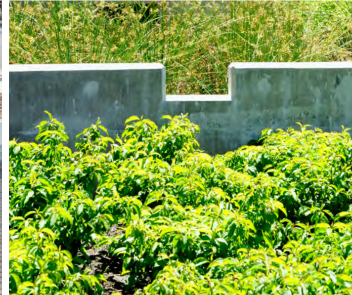
Concrete Planter Walls
