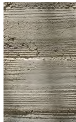
Board-Formed Concrete
