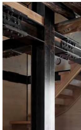
Painted steel structure
