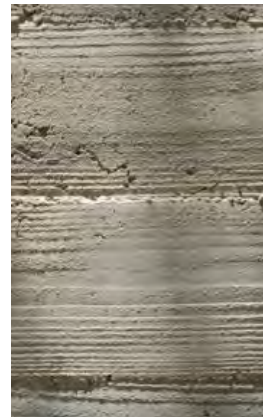
Board-Formed Concrete
