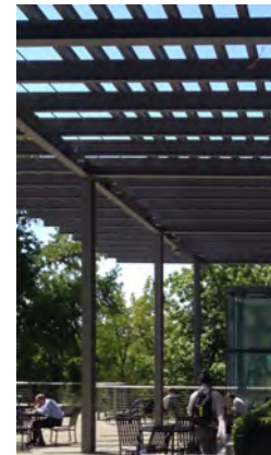
Painted Steel Trellis
