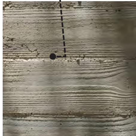
Board - Formed Concrete
