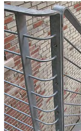
Galvanized rails & roofing
