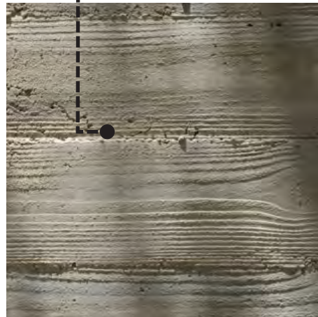
Board - Formed Concrete
