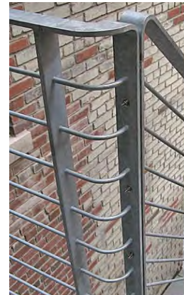
Galv. railing & roofing
