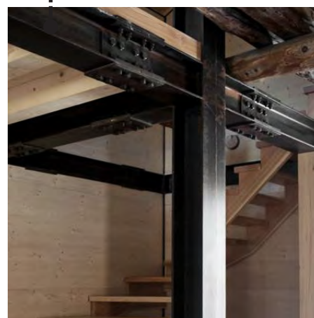
Painted steel structure
