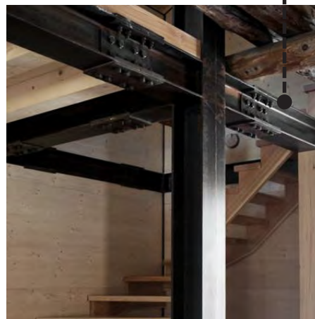
Painted steel structure
