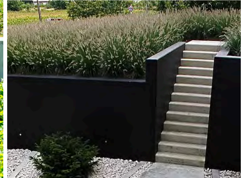
Painted Steel Planter Walls
