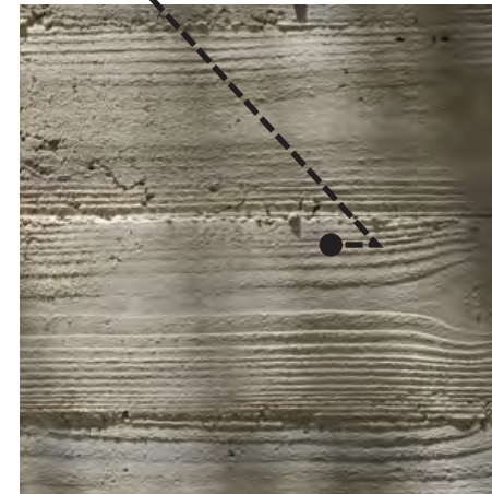
Board - Formed Concrete
