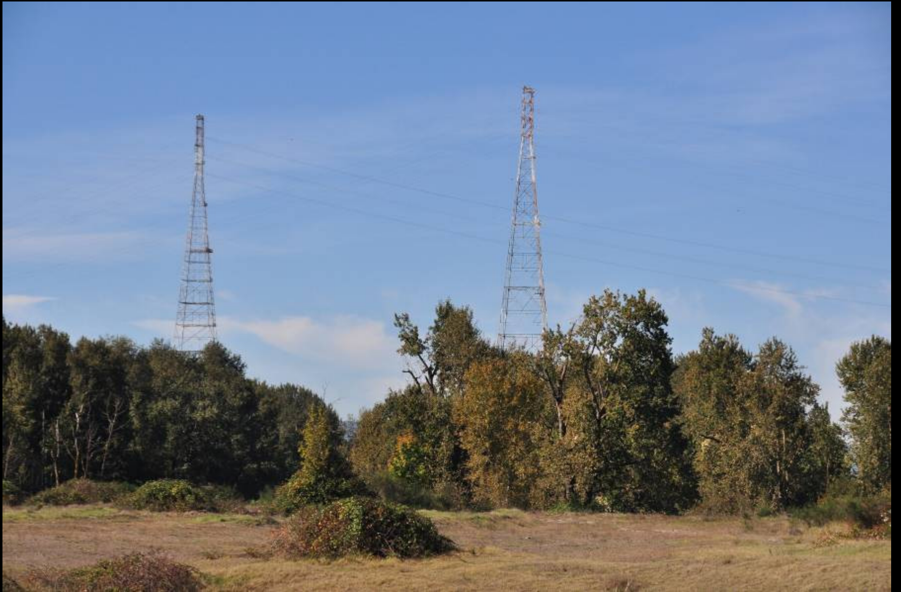
PGE Pylons Carry Power Transmission Lines Across WHI
