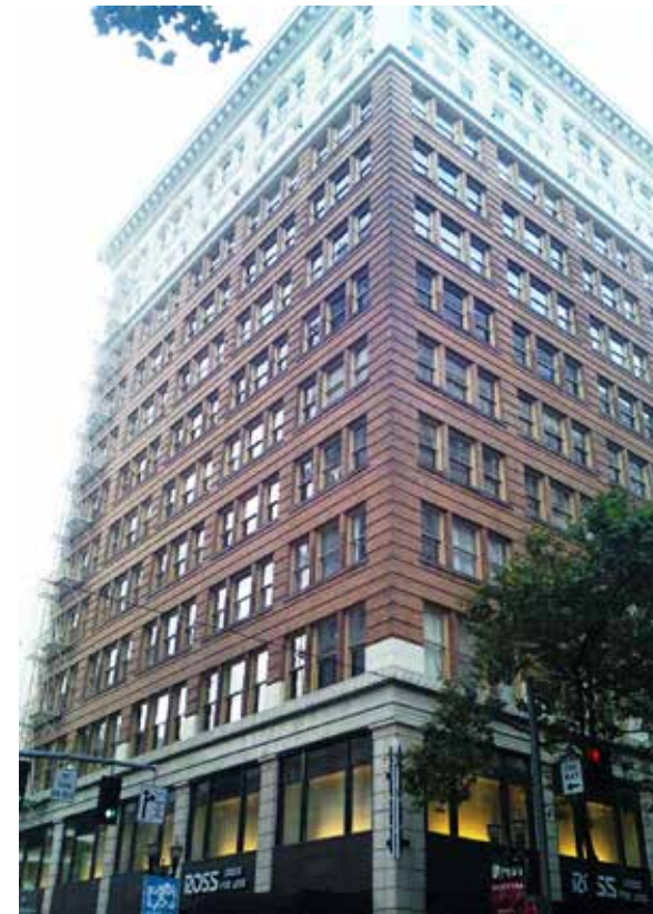
Failing Office Building - 1907
