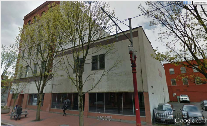
Annex along NW 5th
