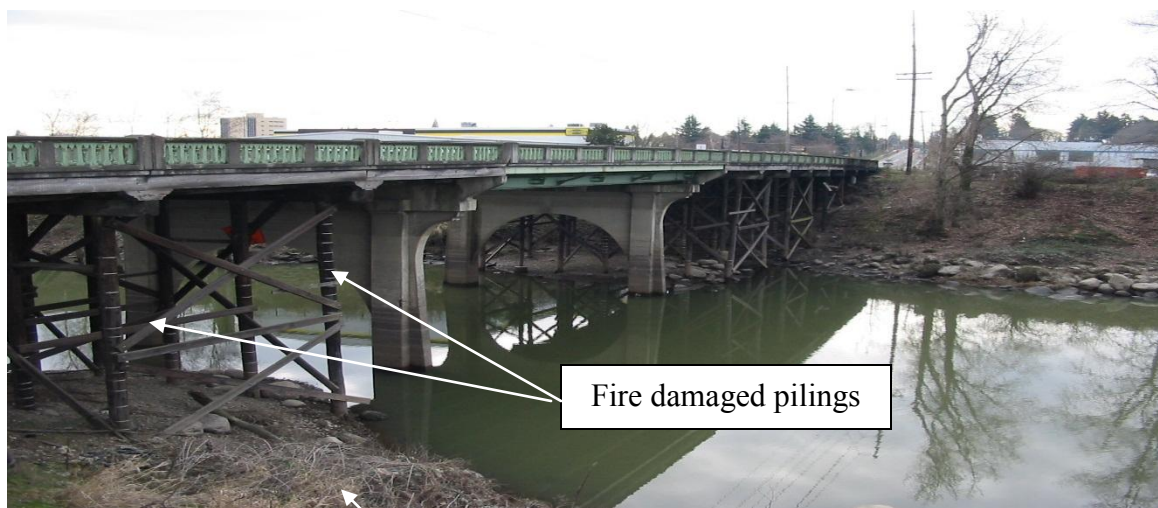
Figure 4. North Vancouver Avenue Bridge before replacement.
