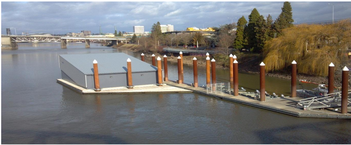
Figure 3. Fire Station 21 Boathouse and Dock
