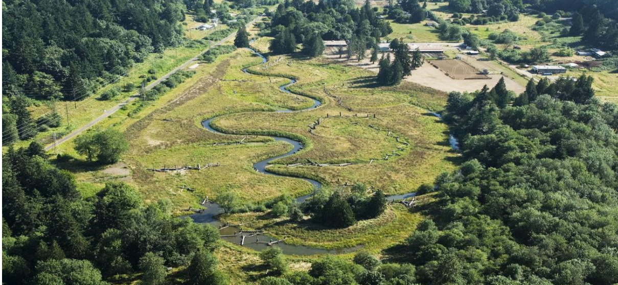
Figure 9. Schweitzer (Brownwood) Natural Area Restoration Project lengthened the channel creating meanders that mimic a more natural system with backwater channels providing high-flow storage and refugia.
