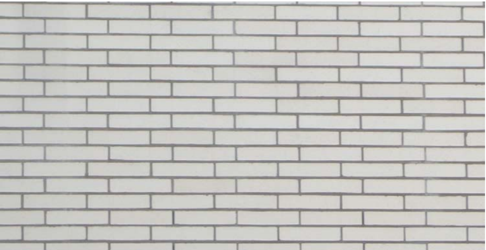
norman size brick 1/3 running bond
