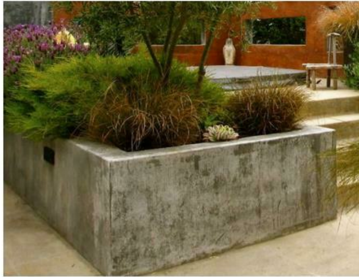
Poured in place raised concrete planters
