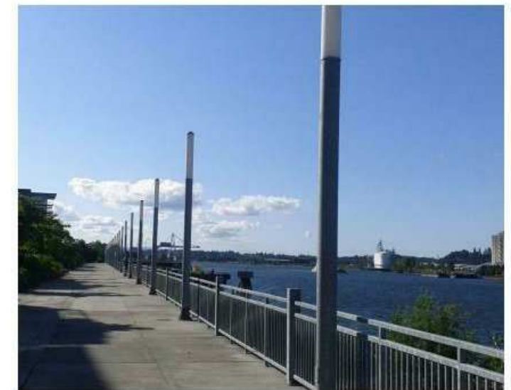
Greenway light fixture
