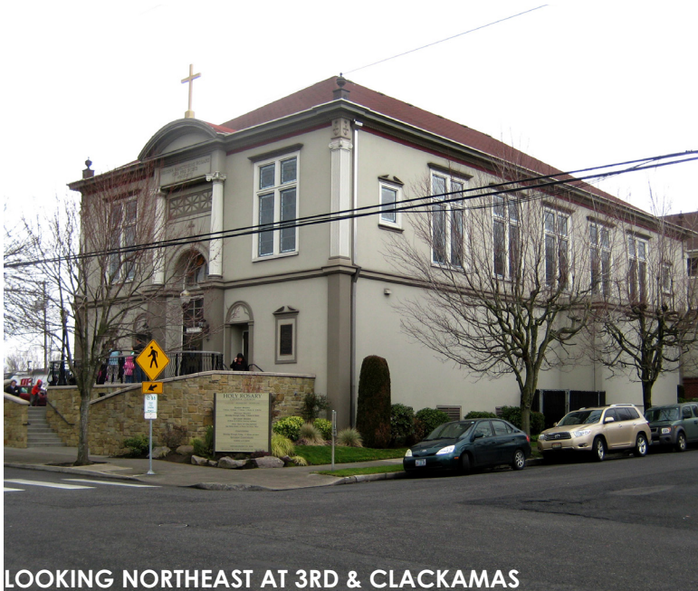
LOOKING NORTHEAST AT 3RD & CLACKAMAS
