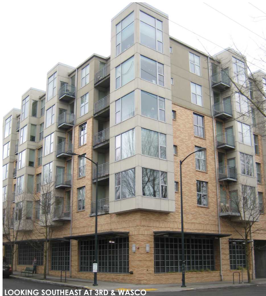
LOOKING SOUTHEAST AT 3RD & WASCO
