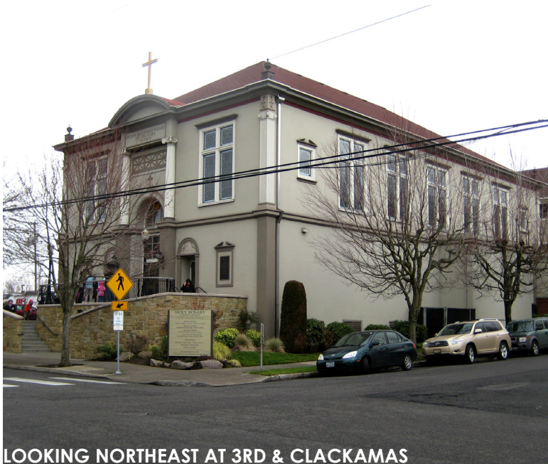
LOOKING NORTHEAST AT 3RD & CLACKAMAS
