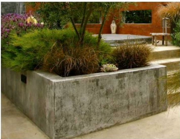
Poured in place raised concrete planters
