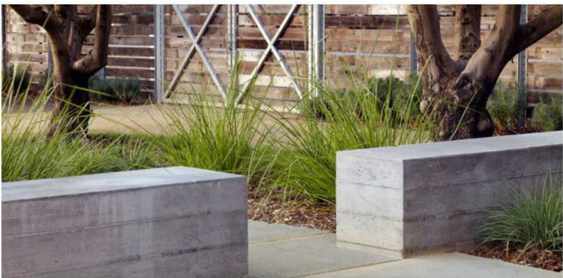
Concrete seatwall benches
