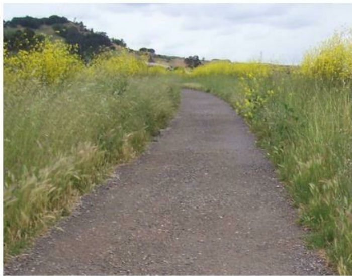
Gravel path at stormwater basin
