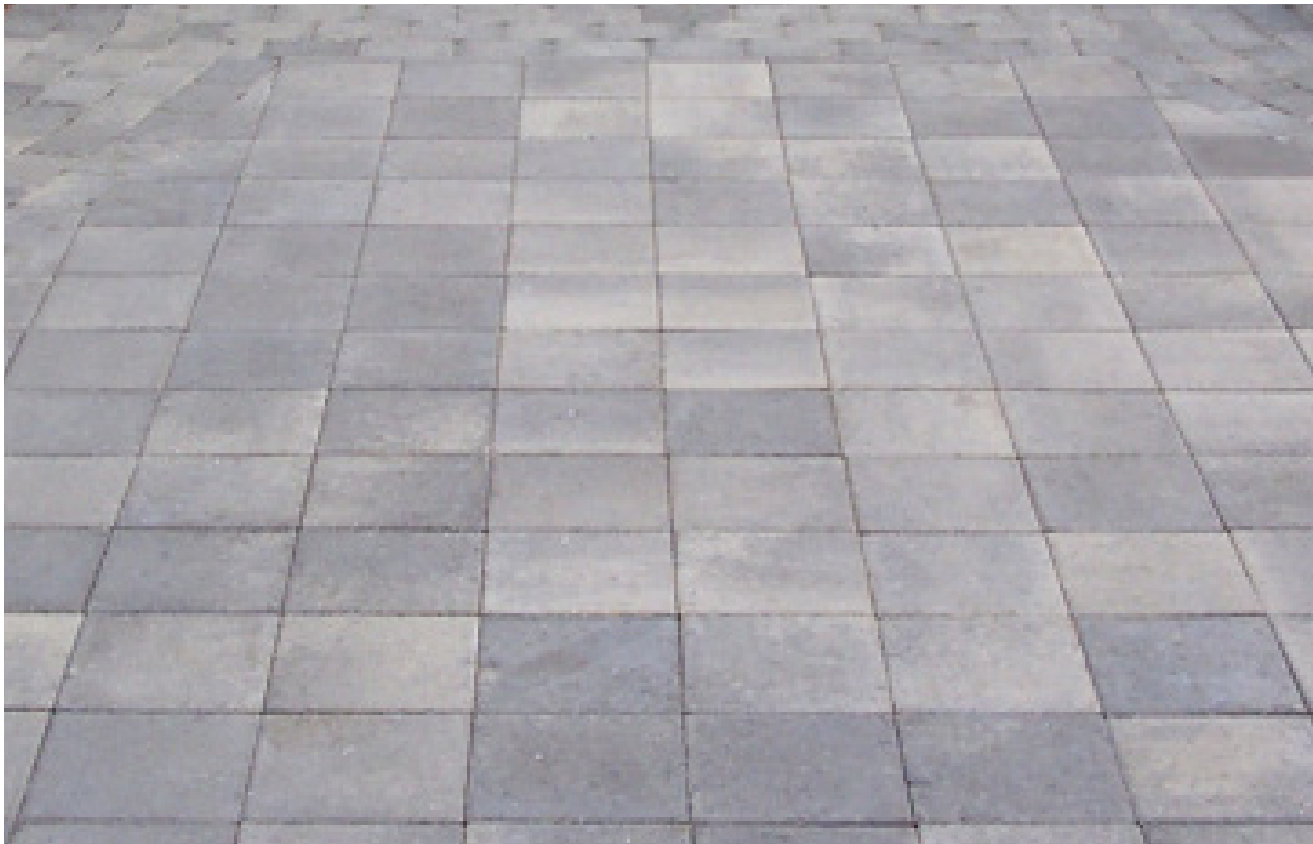
Permeable concrete pavers: Mutual Materials Eco-Prioria
