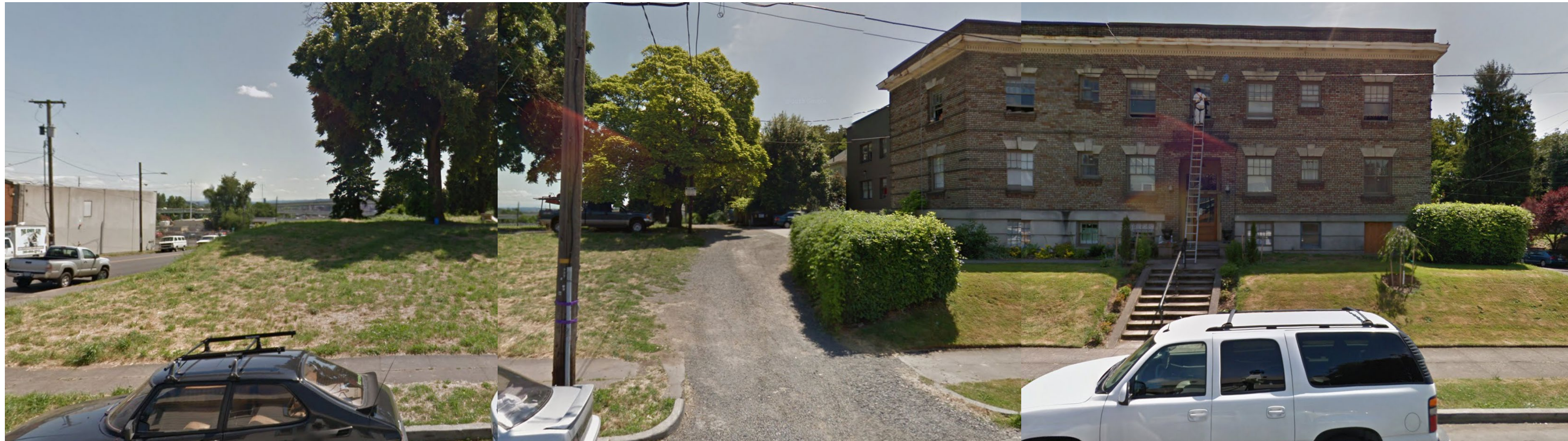
4. View from N Fremont Street
