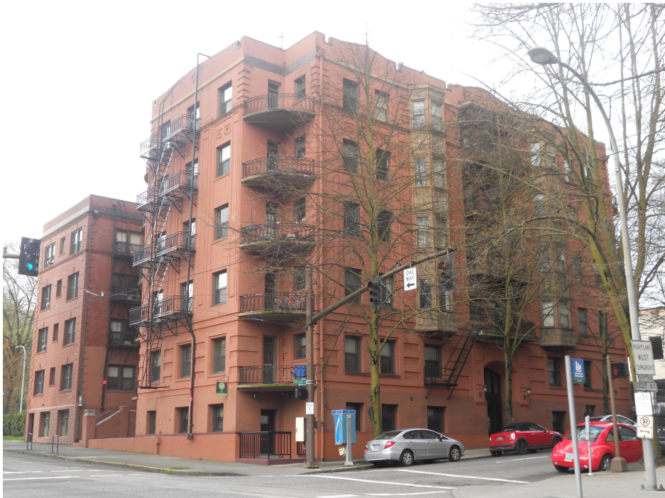
CLAY APARTMENTS 11TH AND CLAY
