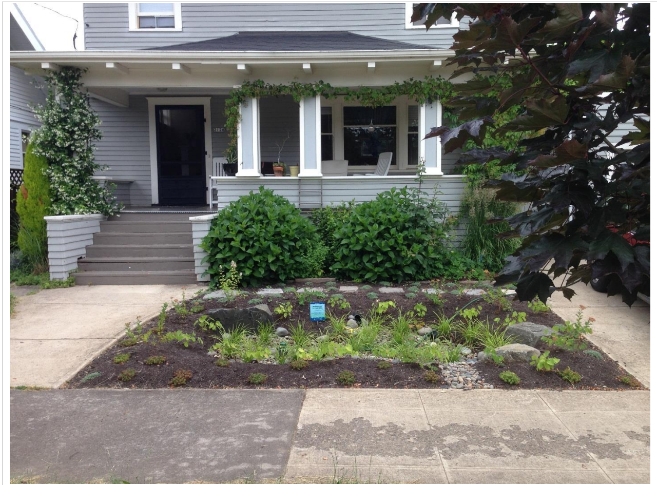
Figure 5-2 Example rain garden, installed in FY 2014
