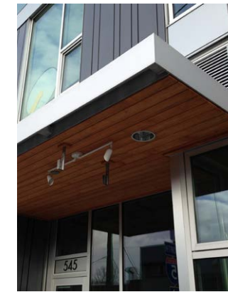
1 STEEL AWNING WITH IPE PLANK SOFFIT
