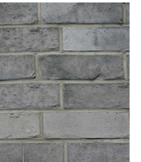
3 CONCRETE MODULAR PAVERS
