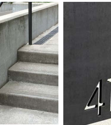
CAST CONCRETE STAIRS
