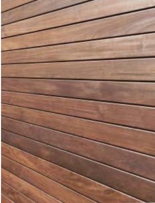
11 IPE PLANK PARTITION SCREEN AND SOFFIT
