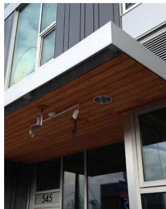
STEEL AWNING WITH IPE PLANK SOFFIT
