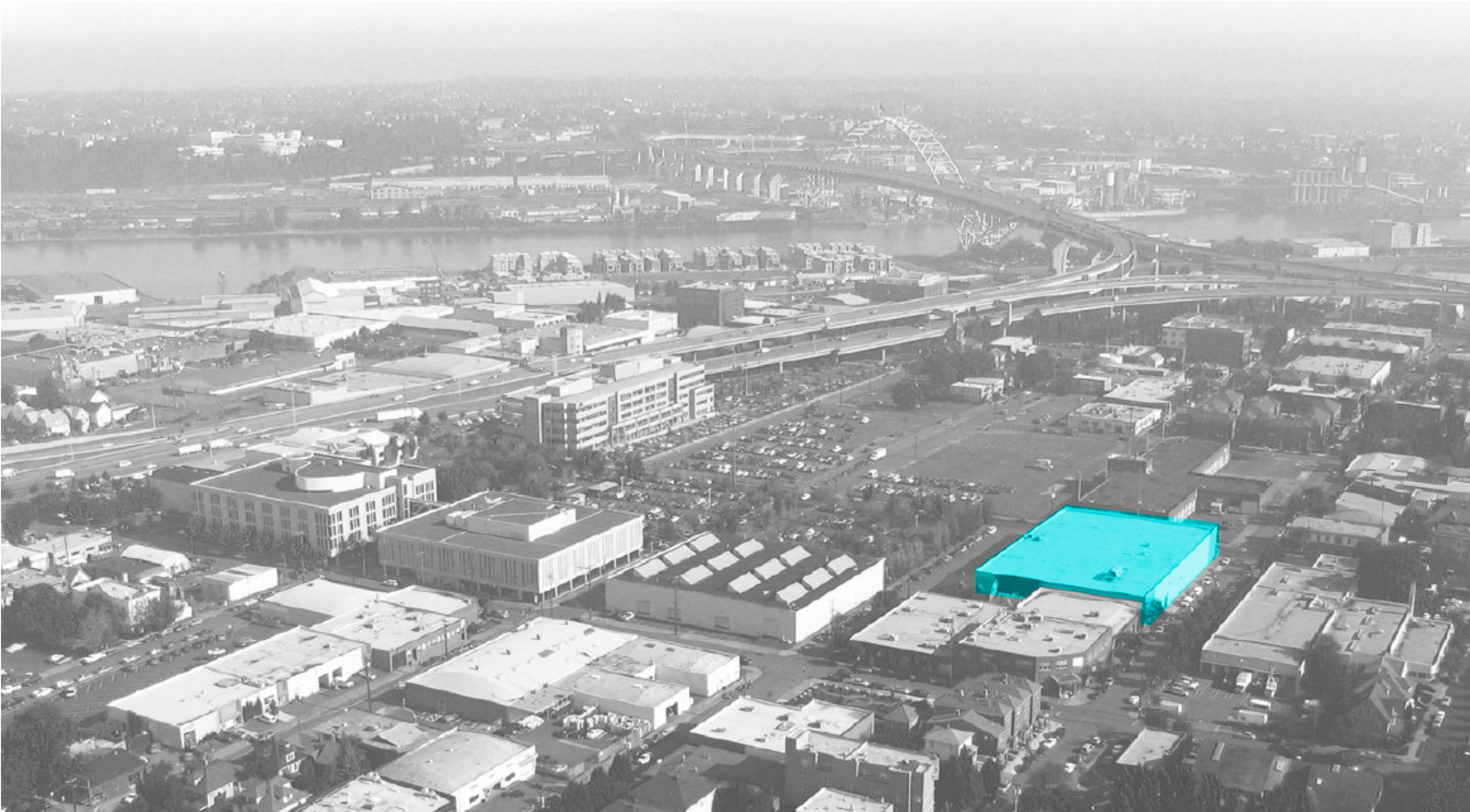
OVERHEAD PHOTO LOOKING NORTHEAST TOWARD THE FREMONT BRIDGE
