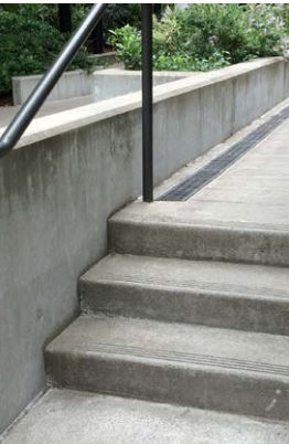
3 CAST CONCRETE STAIRS AND LANDING
