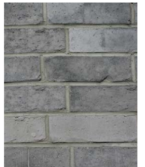
4 CONCRETE MODULAR PAVERS
