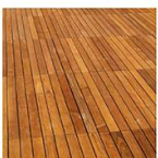
E. Wood Decking
