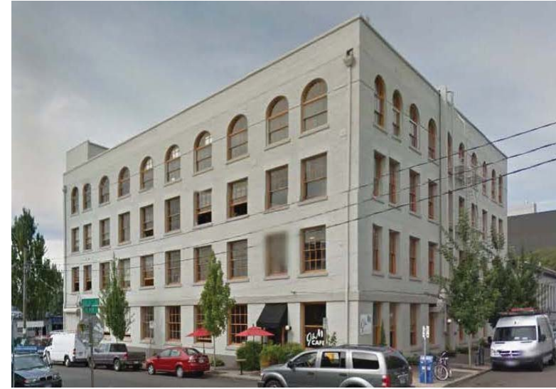
537 SE Ash Street
