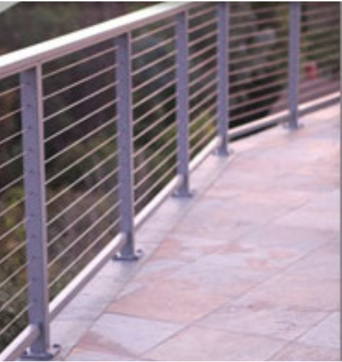
anodized aluminium cable rail
