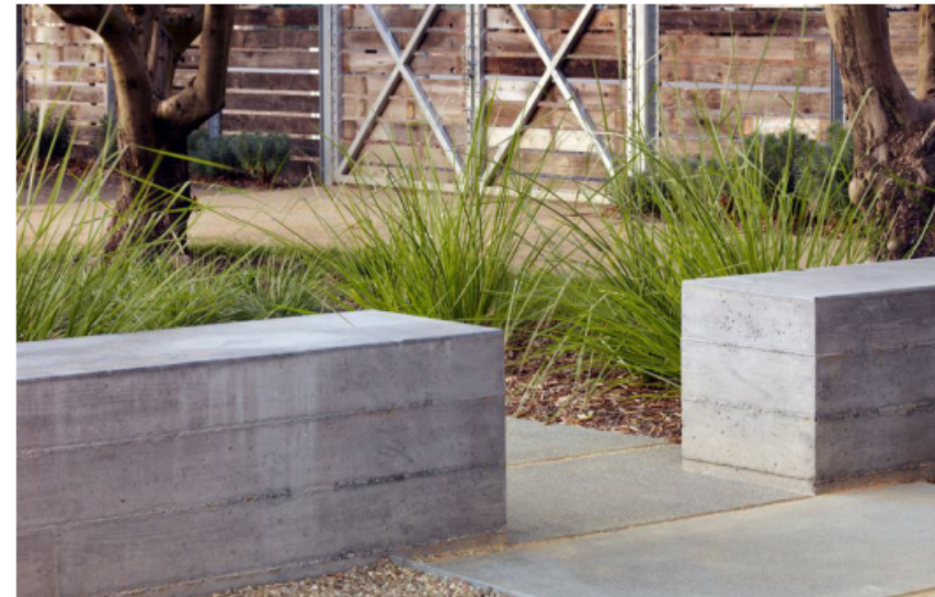
Concrete Seatwall benches
