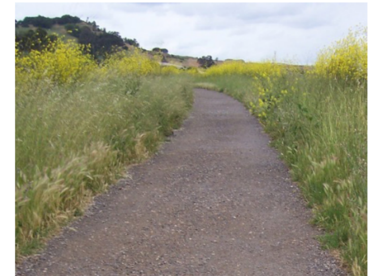
Gravel path at stormwater basin
