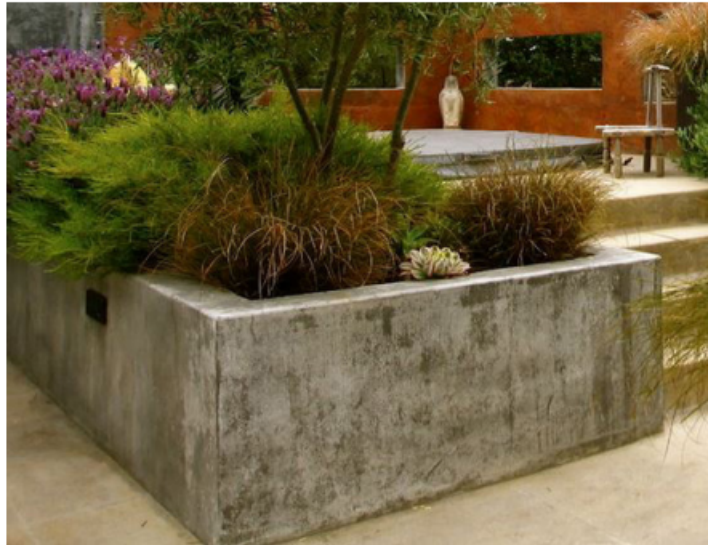
Poured in place raised concrete planters
