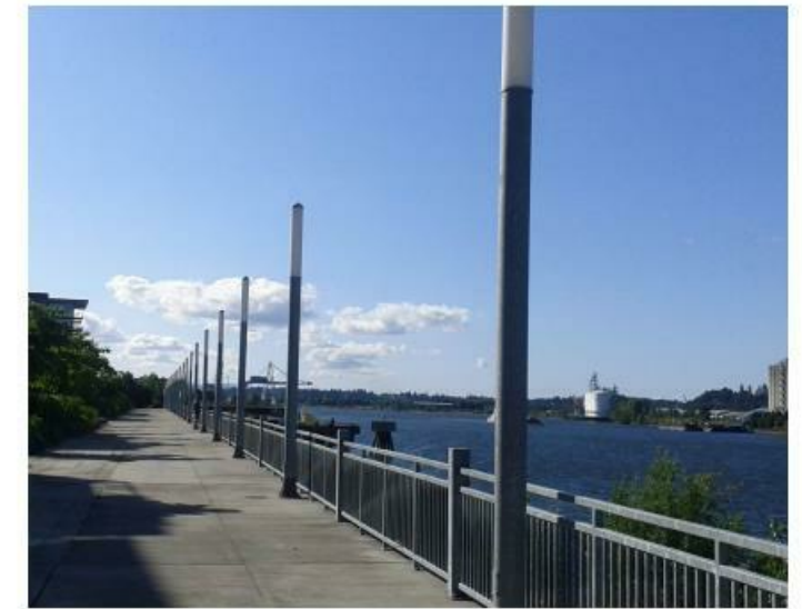
Greenway light fixture
