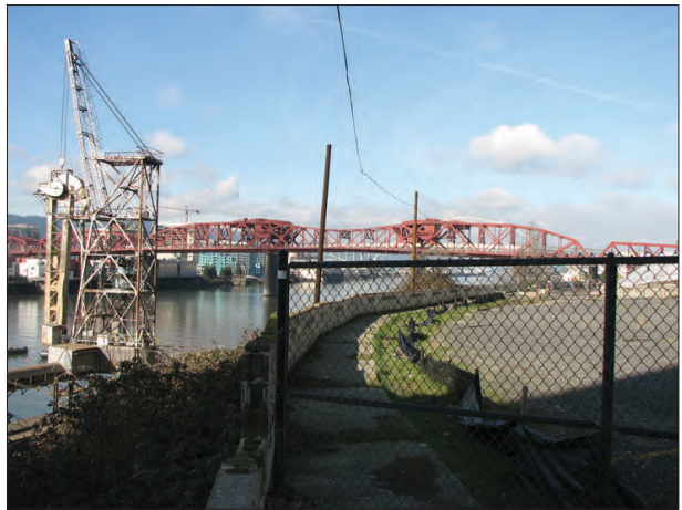
4 N. Dixon streetscape coordination with potential future open space on PPS Blanchard site
