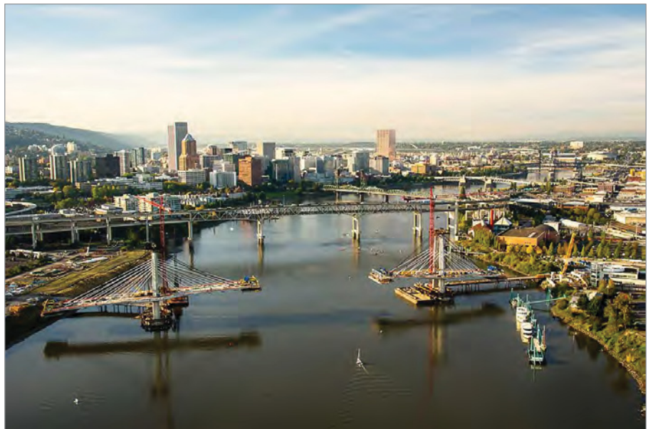
The Tilikum Crossing Bridge under construction, late 2013
