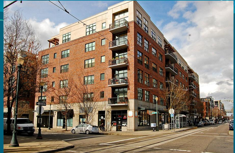
Riverstone Condos (1998) NW 11 th and NW Johnson, looking NW
