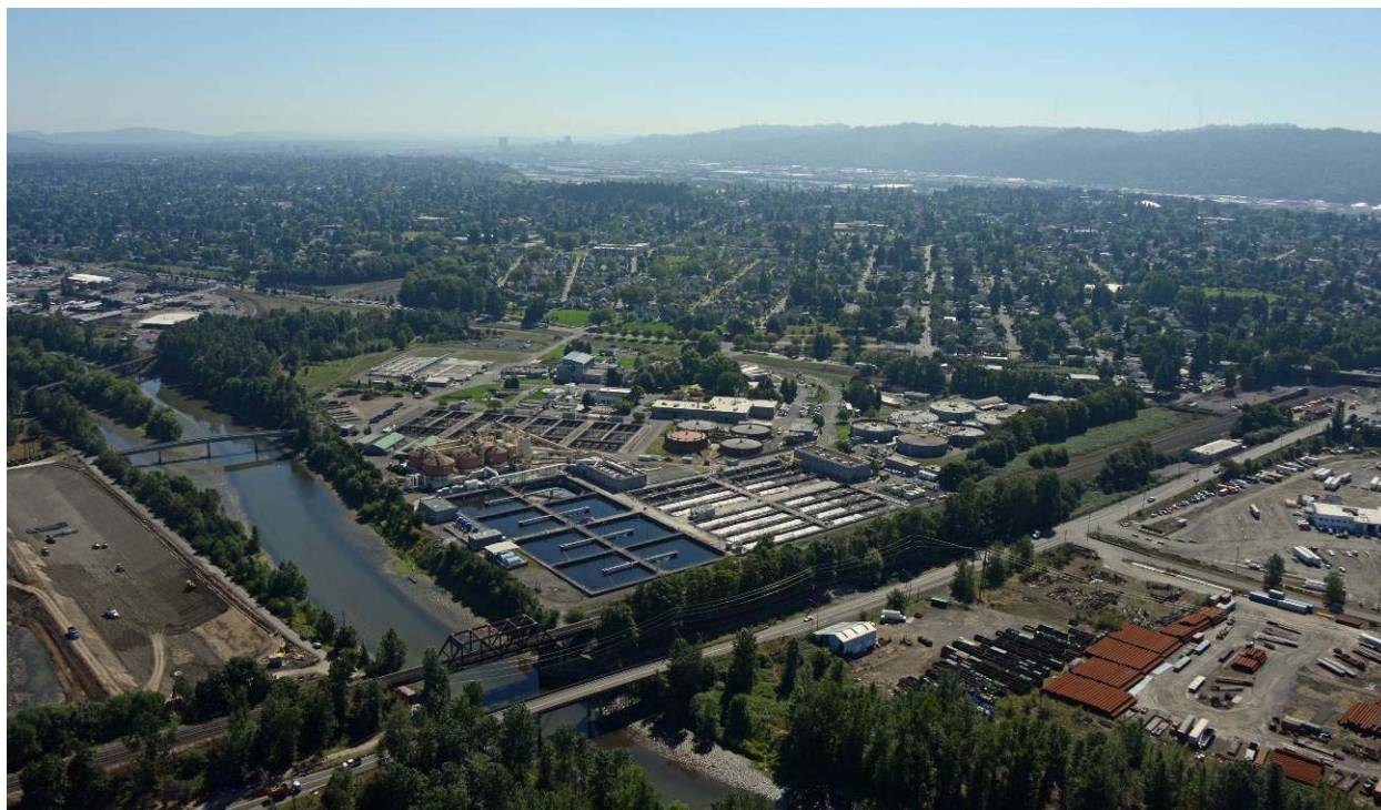
Columbia Boulevard Wastewater Treatment Plant
