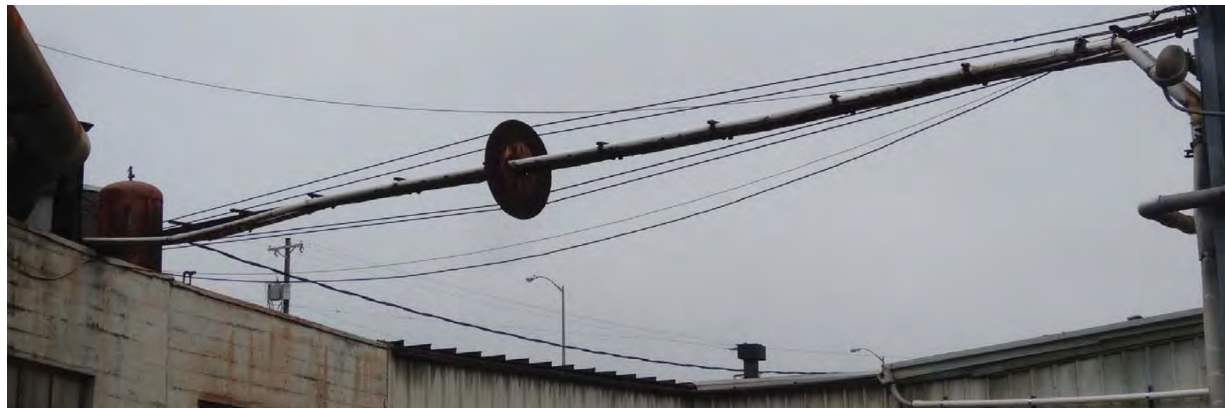
Utility Bridge Structure
