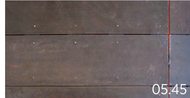
(05.45) NW Elevator Tower Steel Plate Panels w/ Exposed Fasteners
