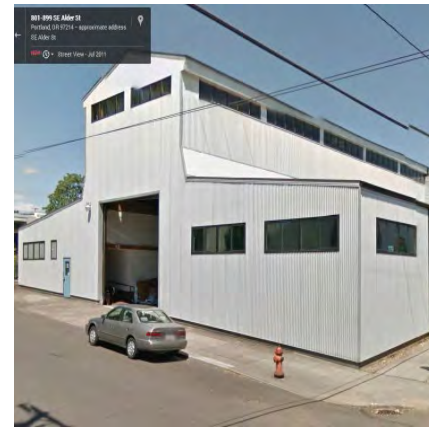
METAL BUILDING NE CORNER OF SE ALDER AND SE 9TH
