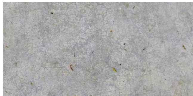
Cast In Place Concrete Base & Planter Walls
