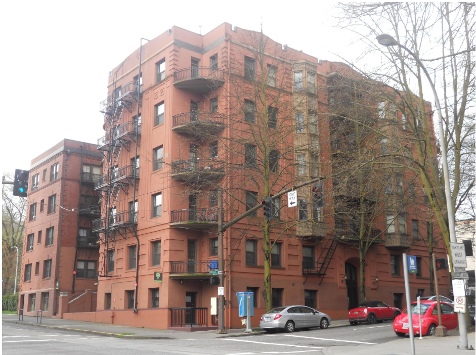
CLAY APARTMENTS 11TH AND CLAY
