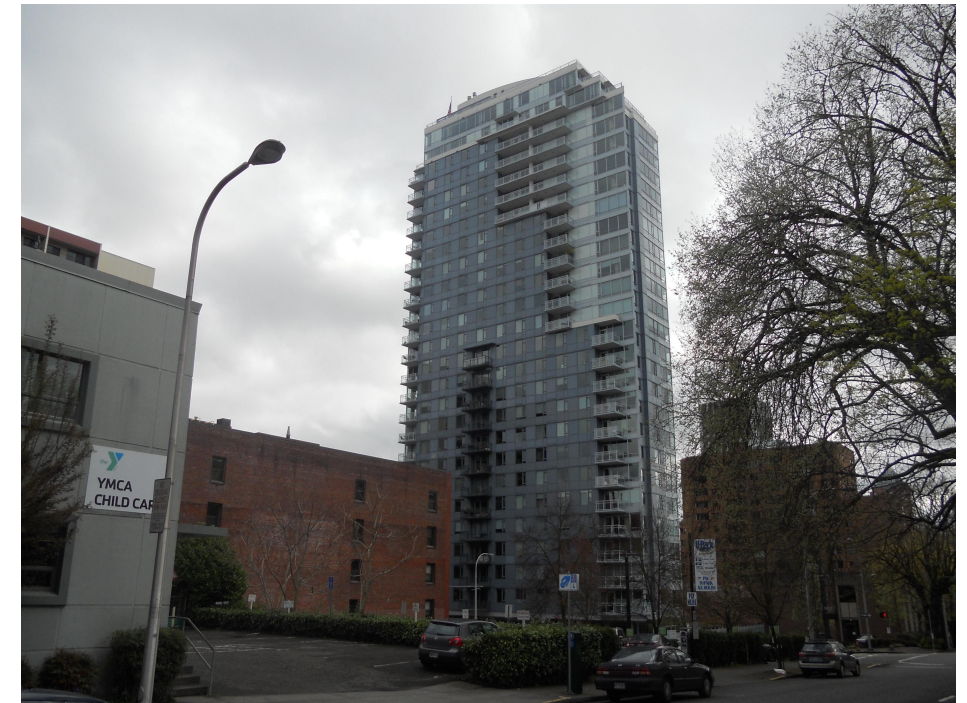
BENSON TOWER 11TH AND CLAY
