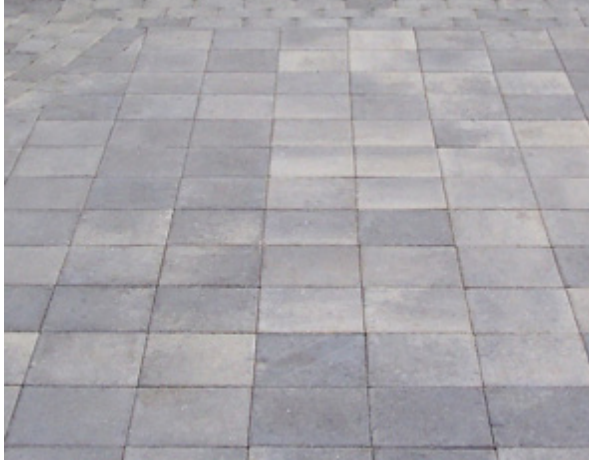
Permeable concrete pavers: Mutual Materials Eco-Prioria
