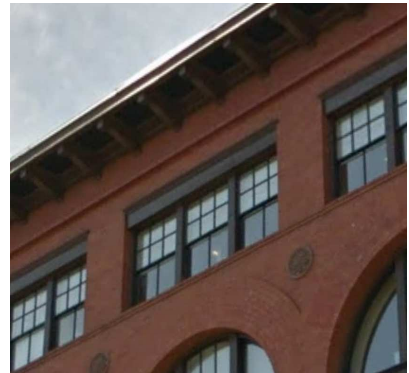
STEEL C-CHANNEL LINTEL ABOVE WINDOWS
