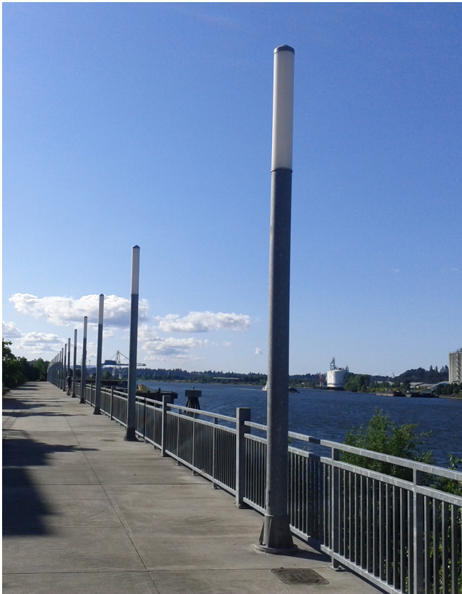
Greenway light fixture
