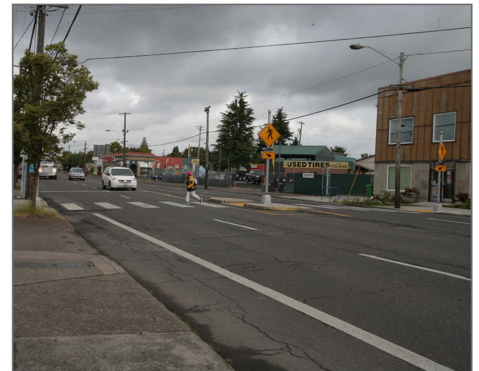
New rectangular rapid flashing beacons (RRFB) improve safety and comfort for people crossing Foster Road.
