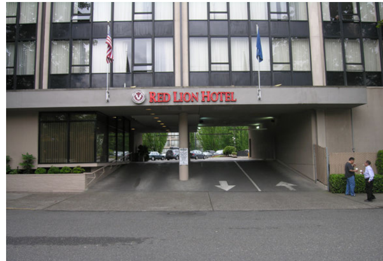
5. View from NE Hassalo St
