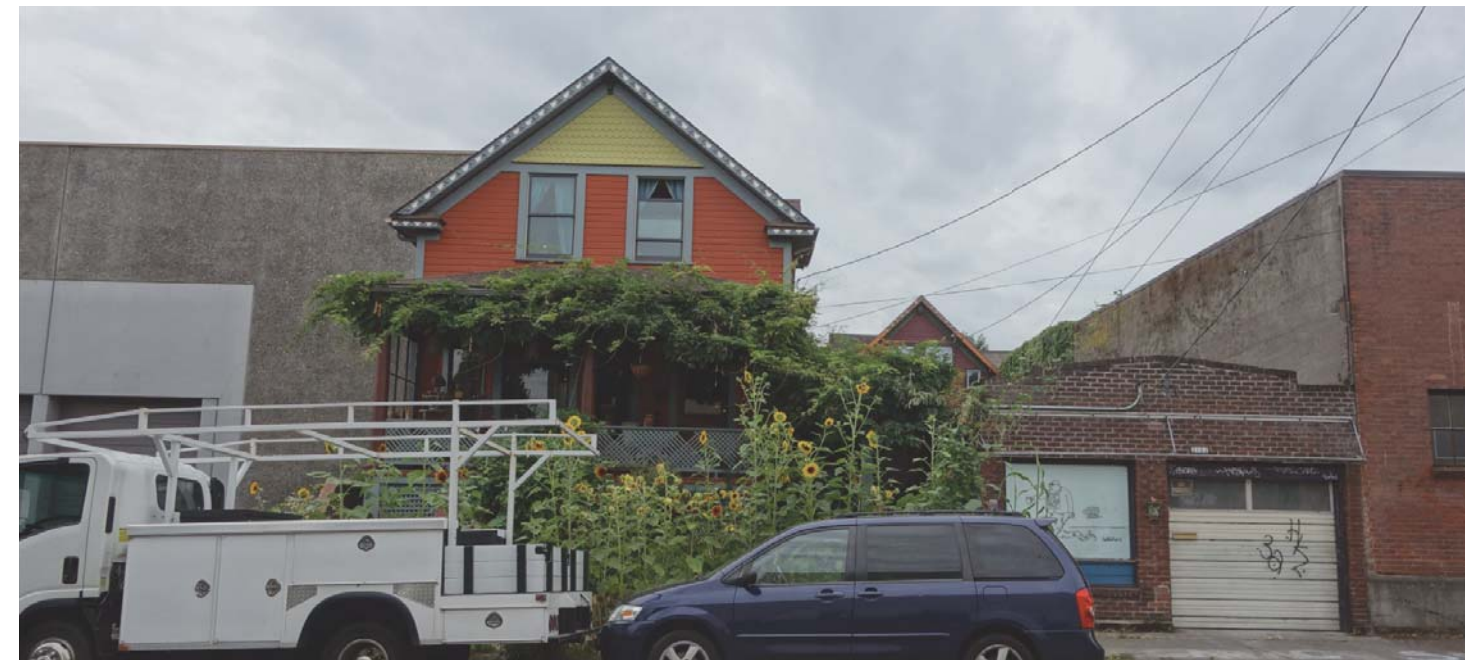
Existing - Quimby St. sidewalk looking South - Existing North facade and neighbor
