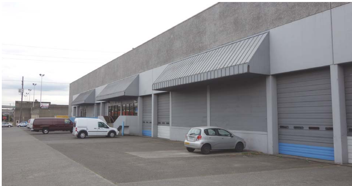
Existing - Quimby St. sidewalk looking East - Existing North Facade
