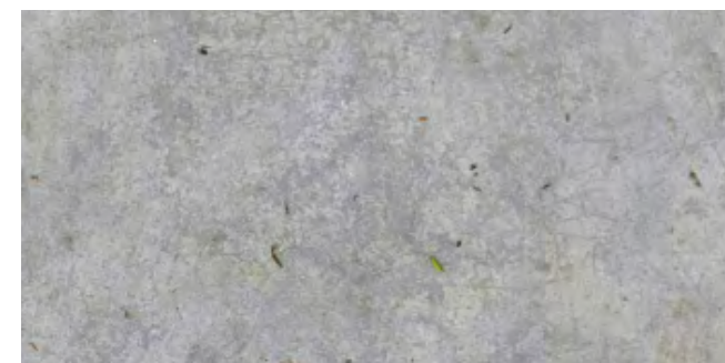
Cast In Place Concrete Base
