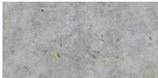
Cast In Place Concrete Base & Planter Walls
