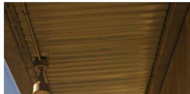
(05.30) Ground Floor Canopies Exposed Roof Decking Galvanized Steel Finish
