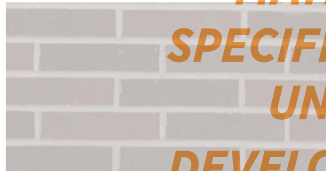
Brick Veneer Color 2 -Mutual Materials Mauna Loa 50% Ebony 50% Mission Texture / Norman Brick
