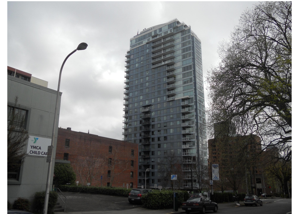
BENSON TOWER 11TH AND CLAY
