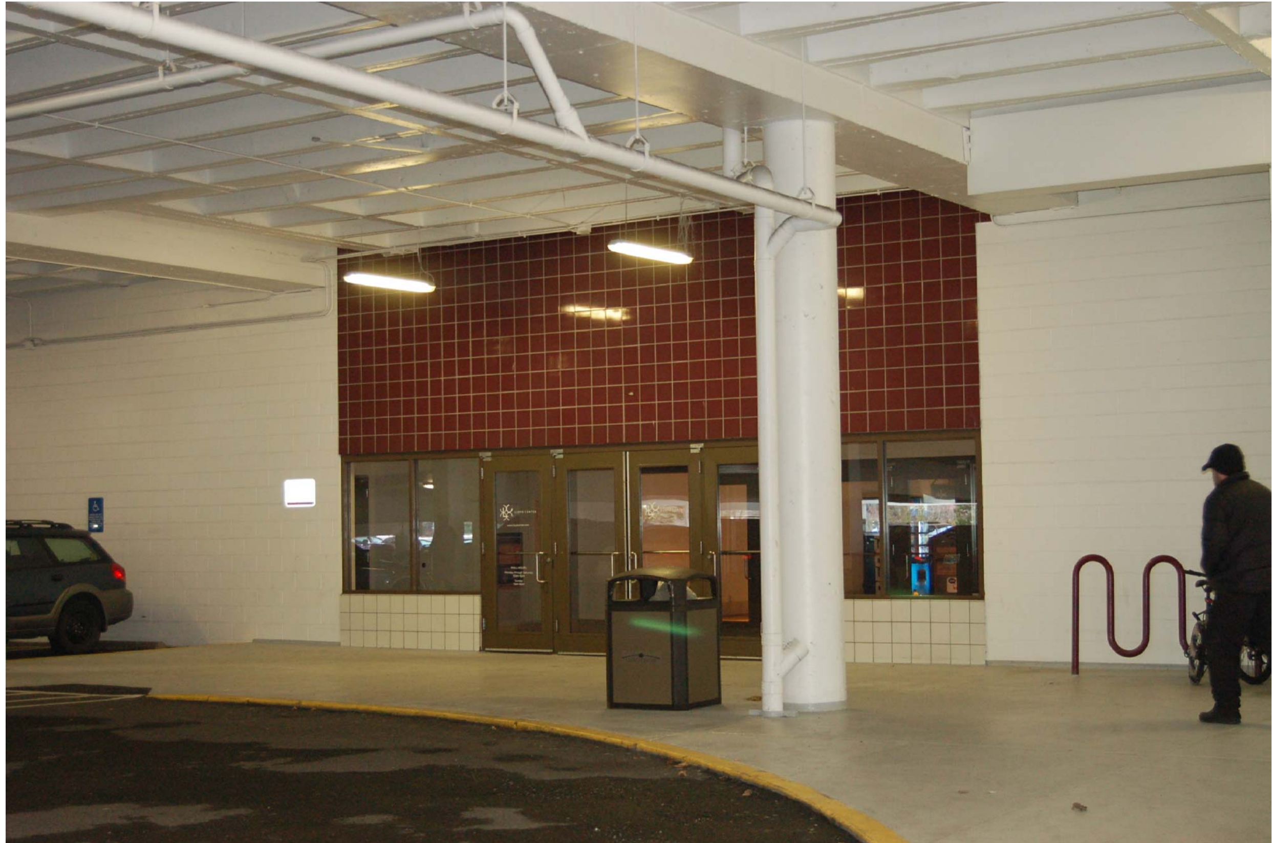
mall entrance from parking existing
