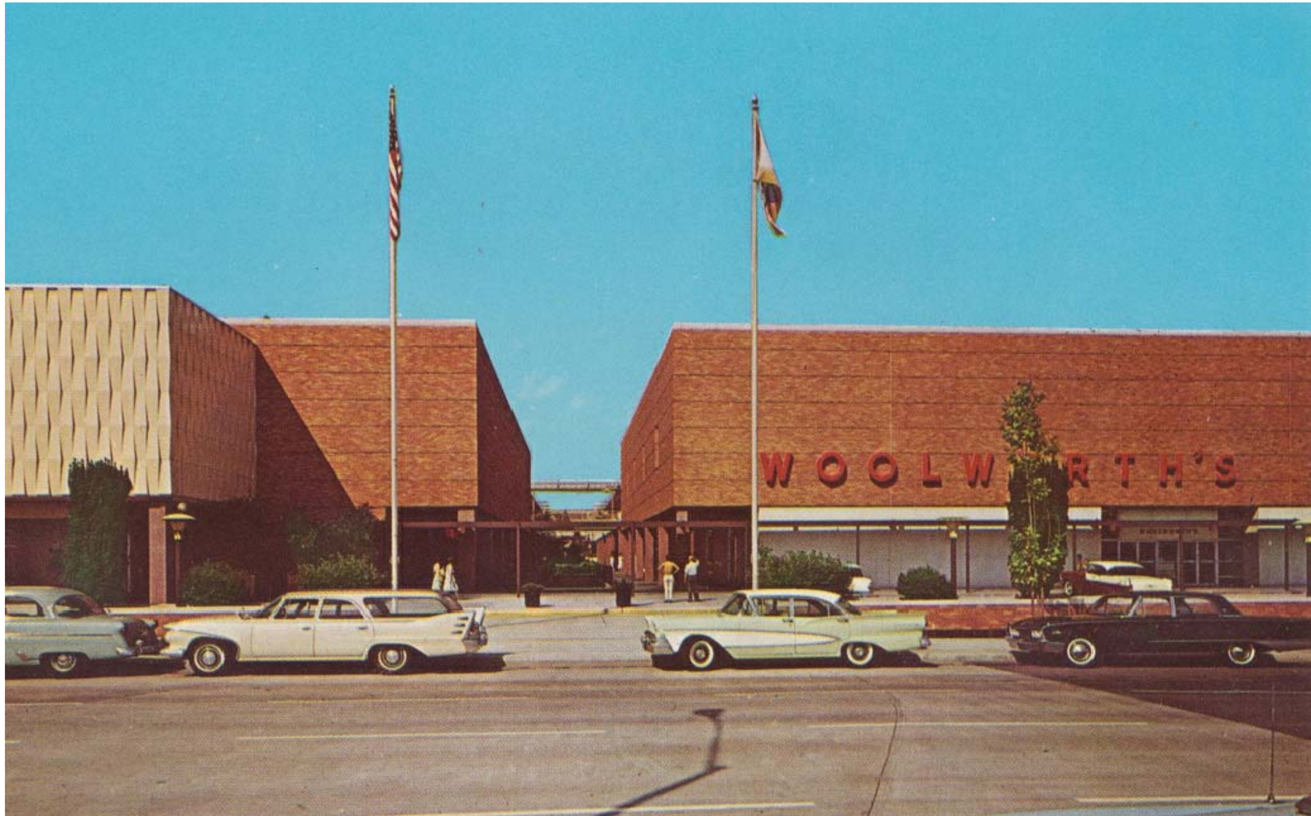
east mall entrance
