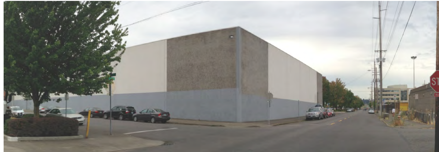
Existing - 21st Street looking Southwest - Existing South and East facades
