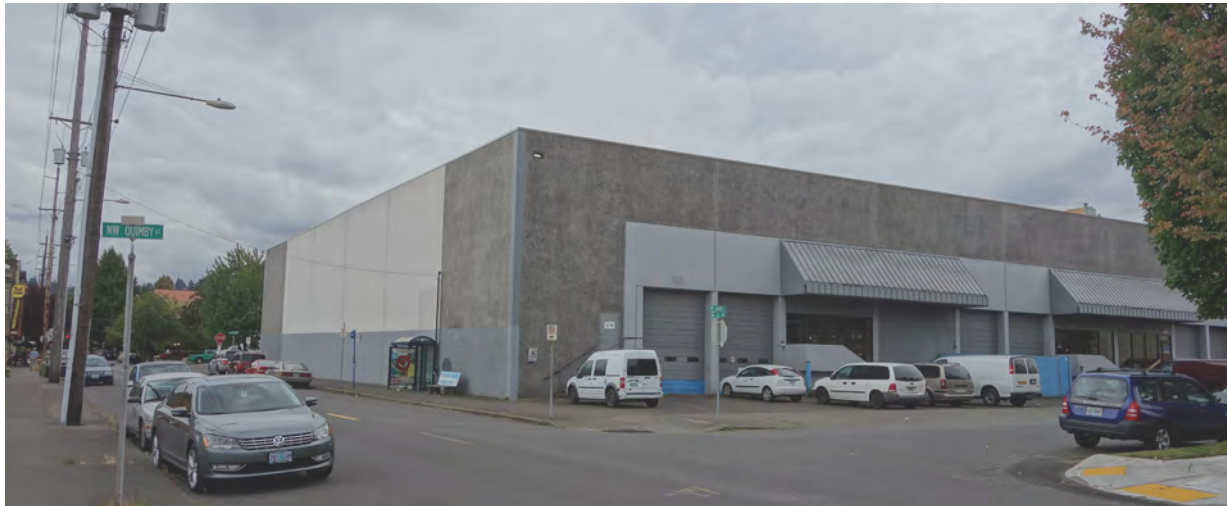
Existing - 21st Street looking South - Existing East and North facades
