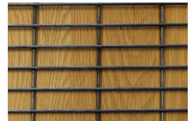
Painted wire mesh guardrail / screen
