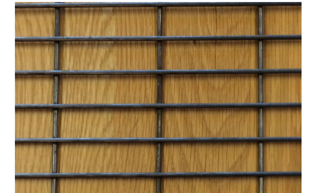
Painted wire mesh guardrail / screen
