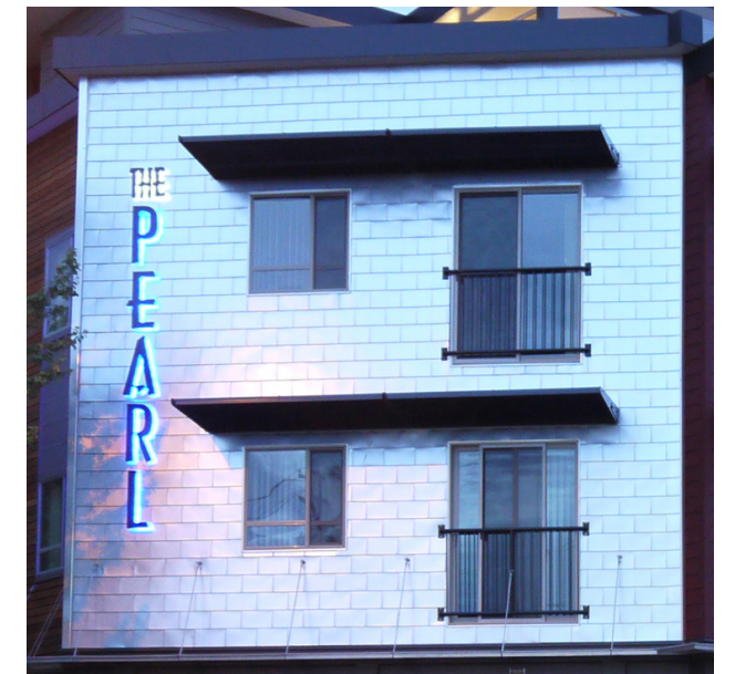
Stainless steel silver tile at upper tower corners
