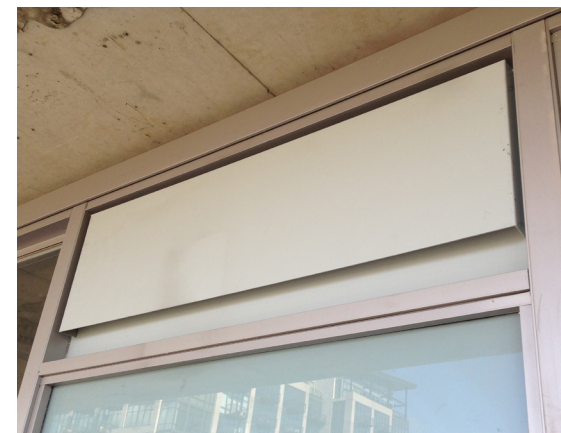
Vented Metal Panel at body and corners
