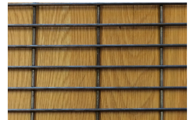
Painted wire mesh guardrail / screen
