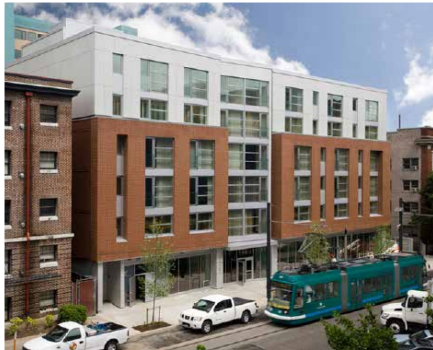
The Jeffery, on the same block, 11th Avenue
