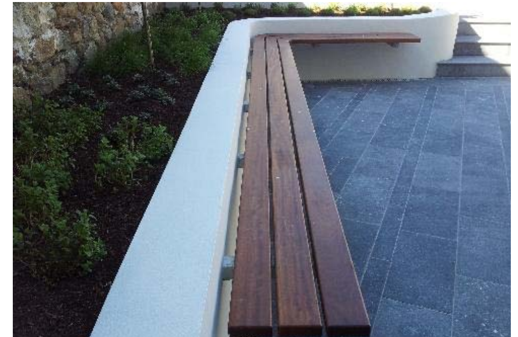
Wood bench mounted to planter wall edge
