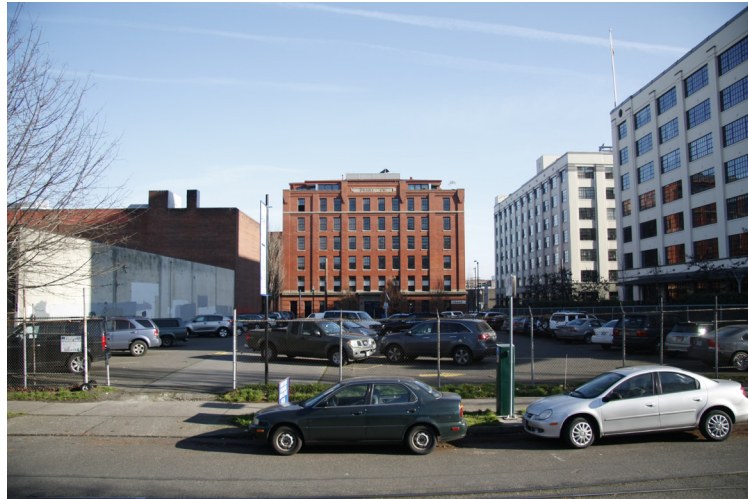
NW 15th Ave. Facing East
