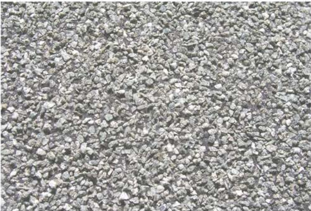
BUILT-UP ASPHALT ROOFING WITH AGGREGATE SURFACING
