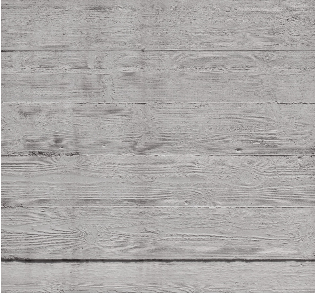
BOARD FORMED CONCRETE
