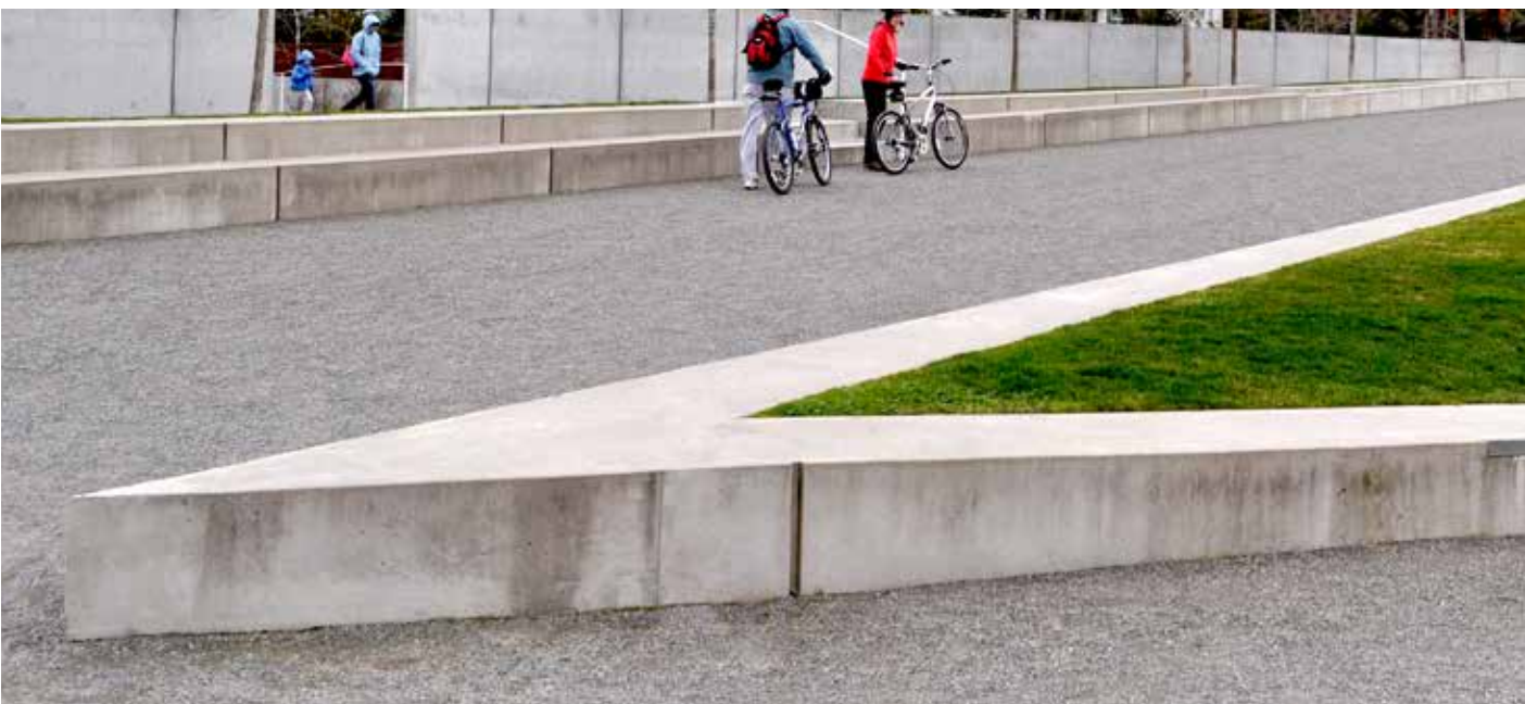
ANGULAR CONCRETE SEATWALL / PLANTER
