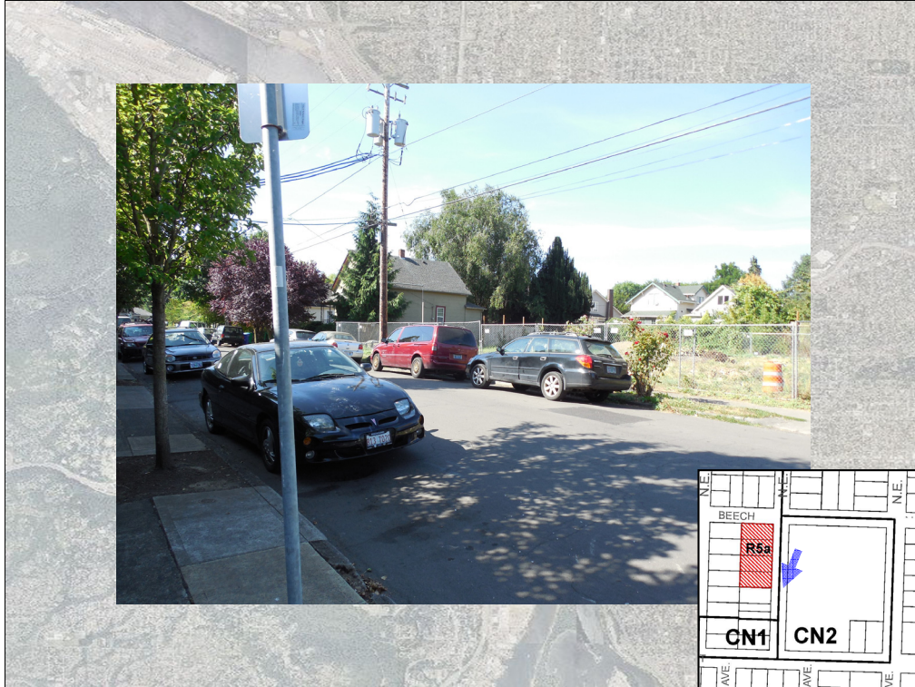
This view is looking south along 14 th avenue toward NE Fremont. The lot immediately south of the 2 vacant lots is developed with a single dwelling home.
